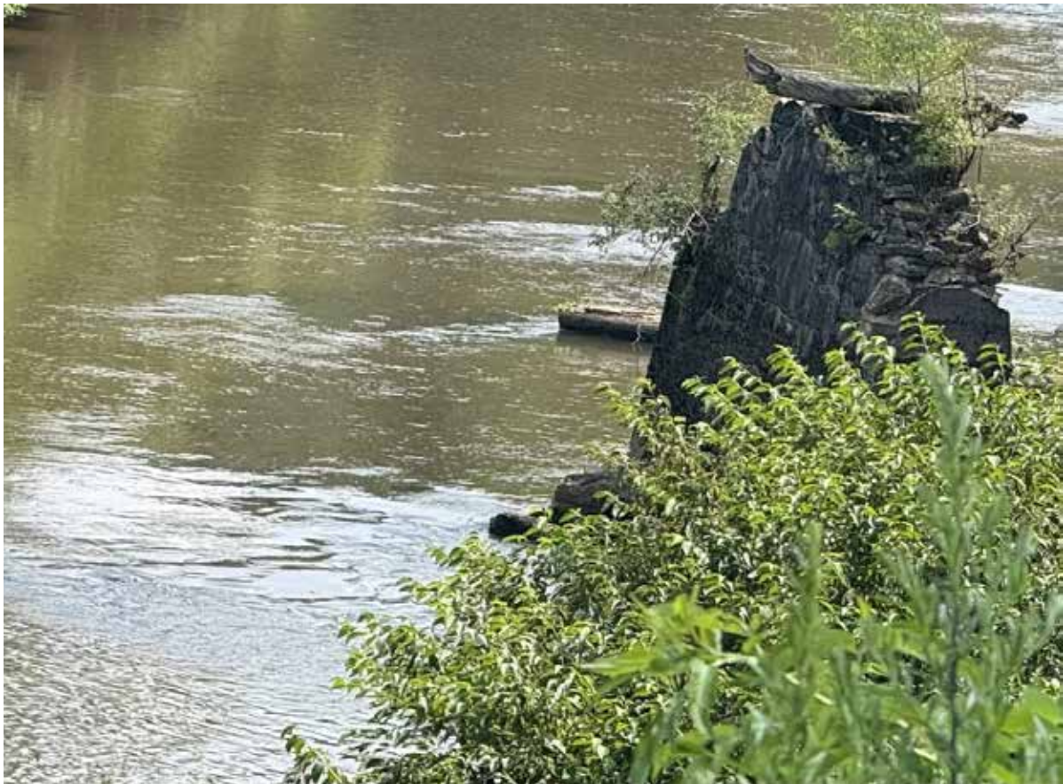
Remnants of the railway bridge as it stands today
